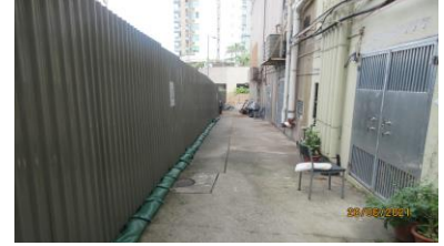
工地豎立圍板 Set-up of site hoarding
